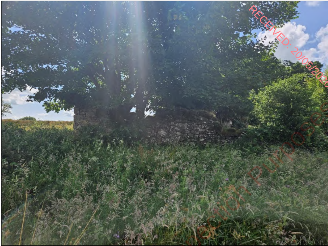
Plate 3-32 Old stone building classified as Stonewalls and other stonework (BL1) located at the southeast of the Site.
