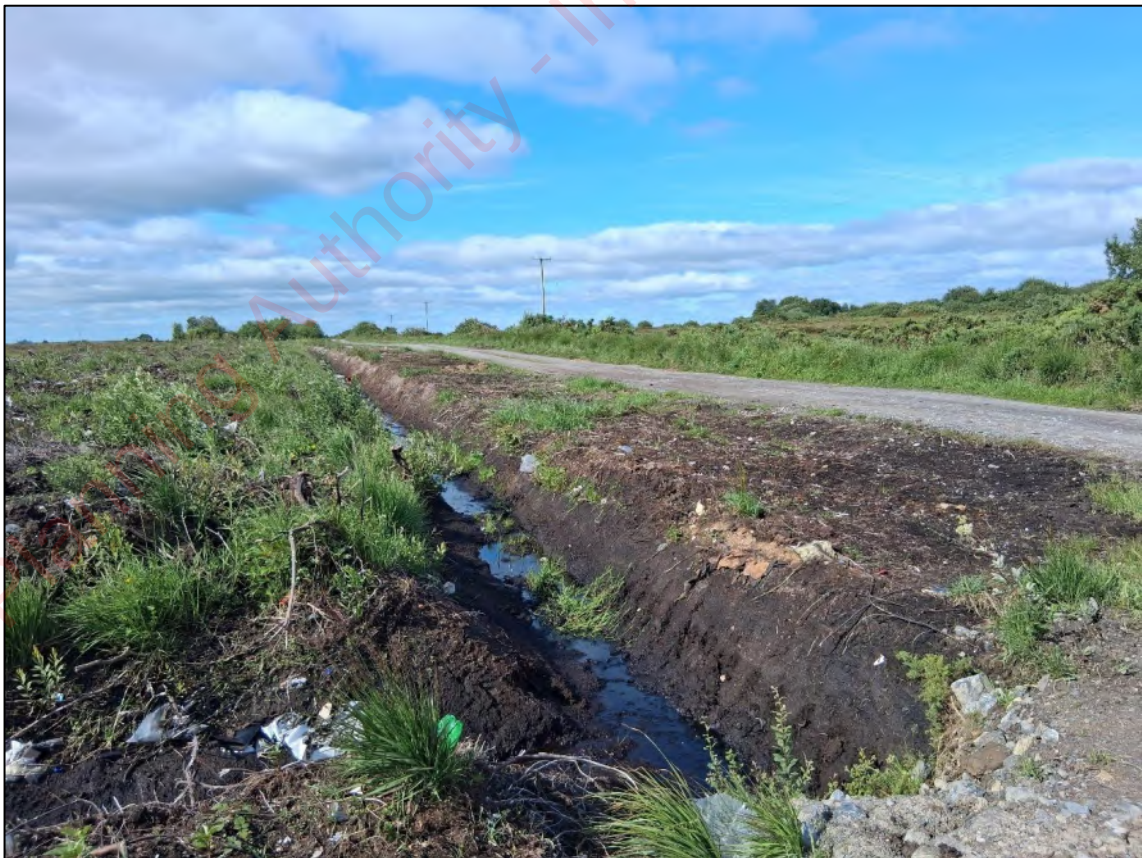
Plate 3-24 A newly-dug Drainage ditch (FW4) within cutover bog habitat in the south of the Site.
